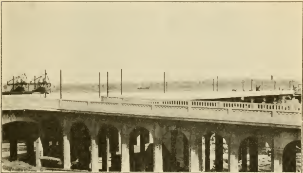
FIG. 10. SECTION 5. SECTION 4 IN BACKGROUND.
